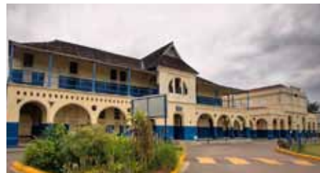
The Scotland Building
