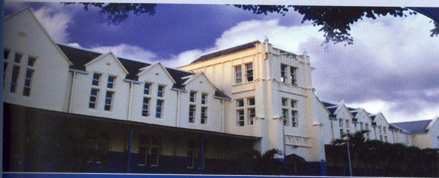
The Simms Building
